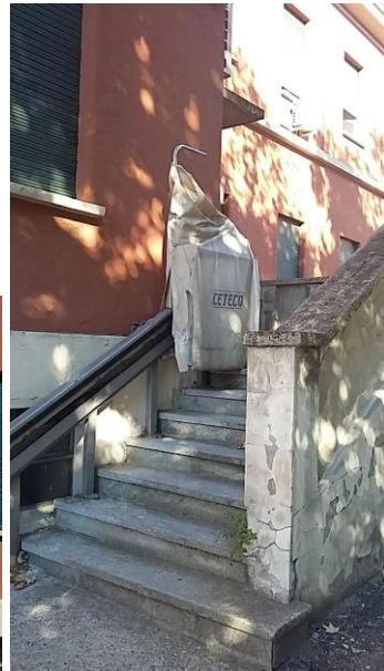
Side entrance of Aula A
