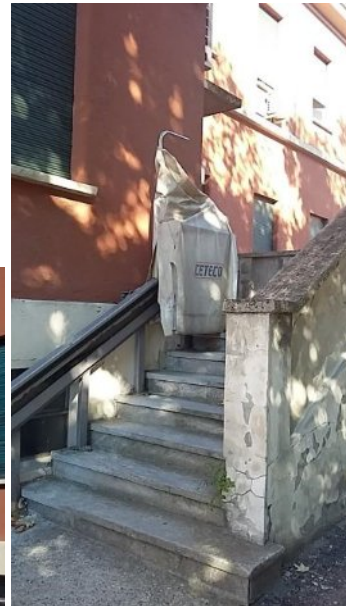
Side entrance of Aula A
